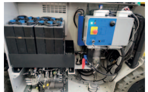
Control box and main battery pack
